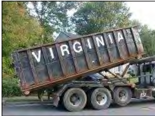
PDS arrives promptly at 8:00am with the first of 2 dumpsters!
